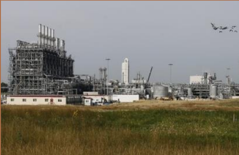
Dow Chemicals, ethylene plant expansion Fort Saskatchewan
