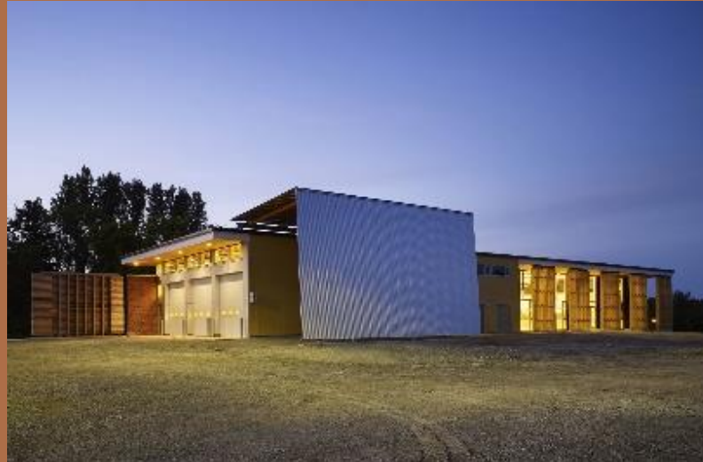
TRCA Restoration Services Building Vaughan, Ontario
